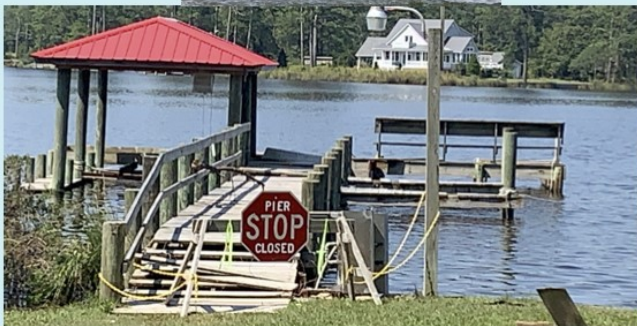
HURRICANE DORIAN DEVASTATED OUR PIER
